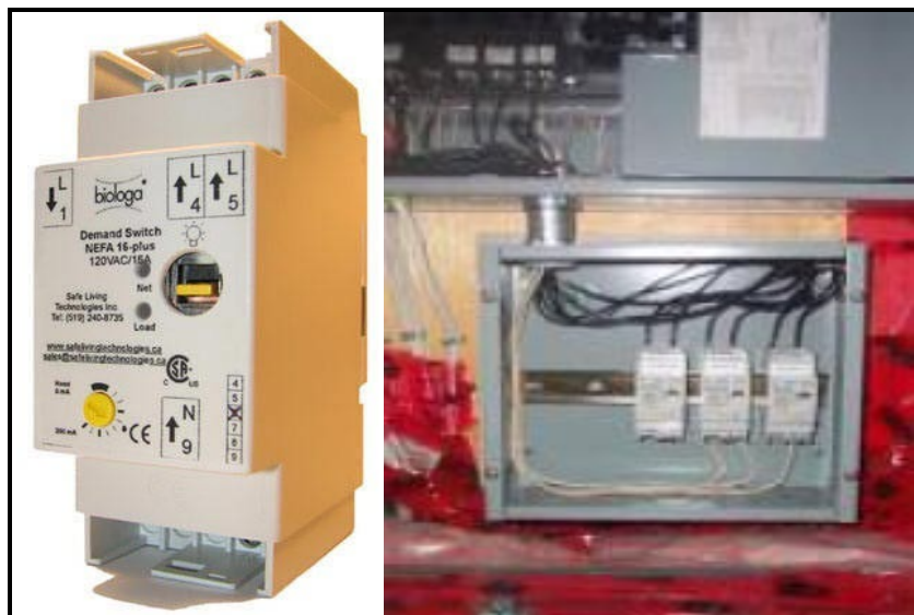
Figure 2.15: Demand switch (left) and installation of demand switches next to the electrical panel (right).
