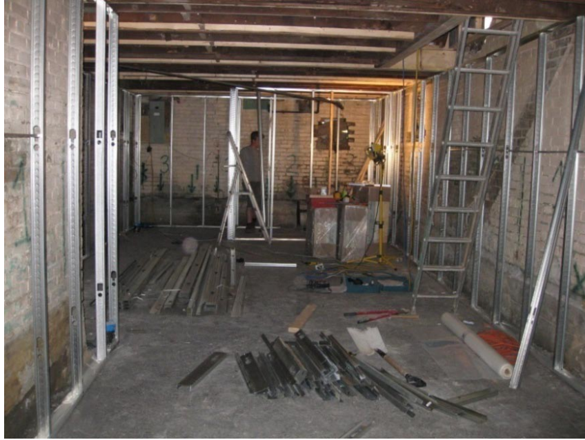
Photo 3: Steel stud framing in the basement.
